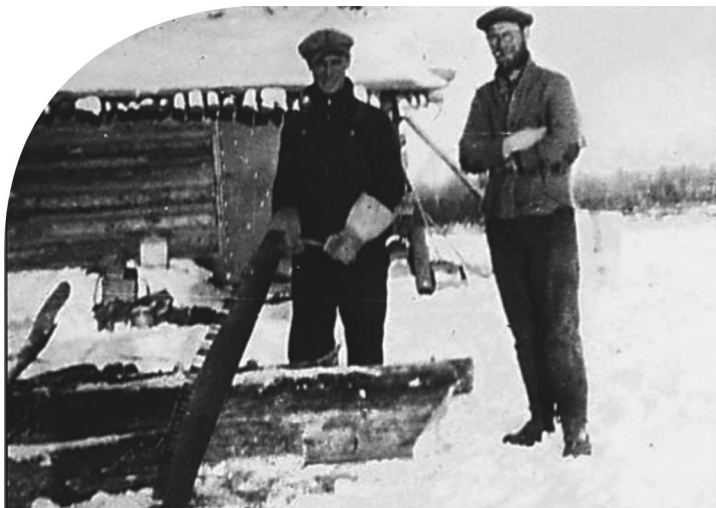
JACK & HARVEY PARKER CUTTING LOGS FOR THE HOUSE
